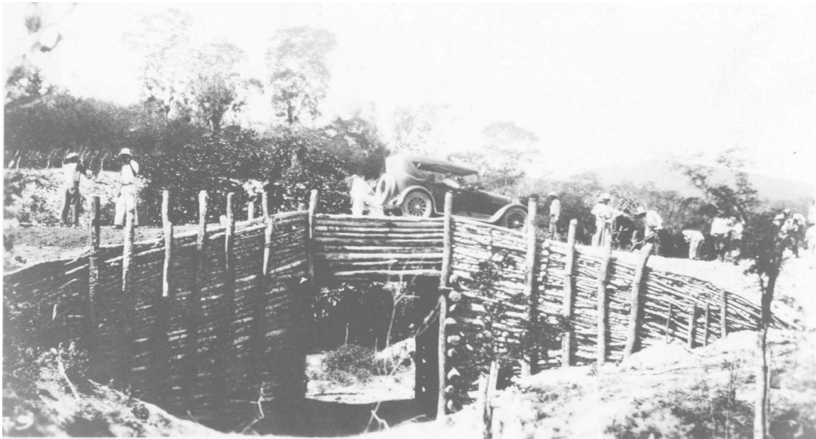
Figure 3-2. Standard military crib bridge. 38
