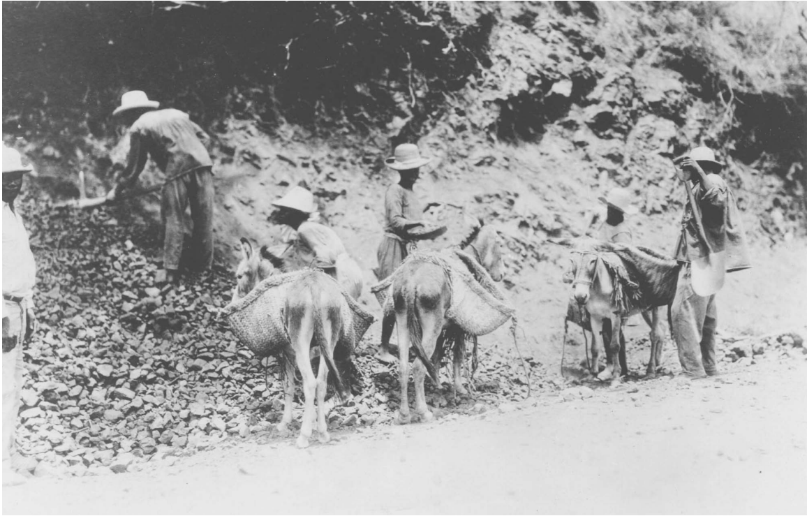
Figure 3-1. Haitian laborers using burros to transport gravel for road resurfacing. 31
