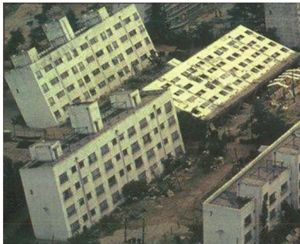
Fig. 9.9 Kawagishi-cho apartment buildings tilt in Japan (adapted from www.ce.washington.edu/.../niigata/niigata.html )
