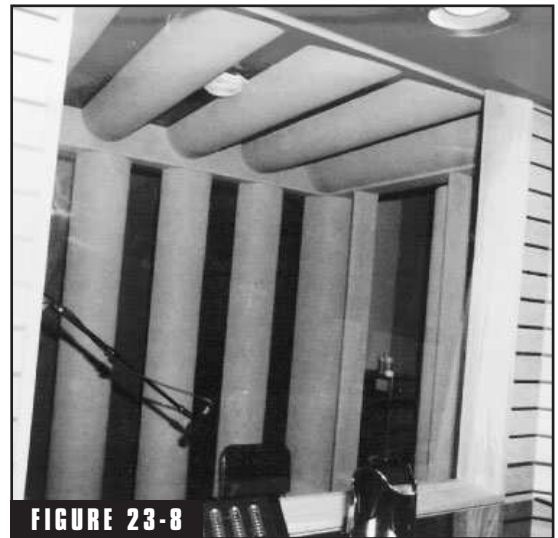
FIGURE 23-8 A studio constructed according to the Quick Sound Field™ principles. (Tube Traps™ have been removed from the window for the photograph.) Acoustic Sciences Corporation.
