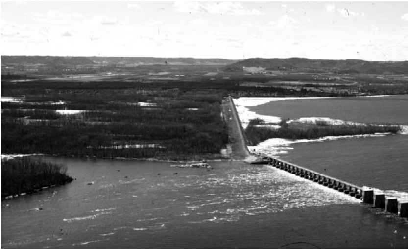
2.9. Lock and Dam 9 at Lynxville showing natural forested island floodplain below the dam to the left and inundated/eroded bottomland above the dam to the right.
