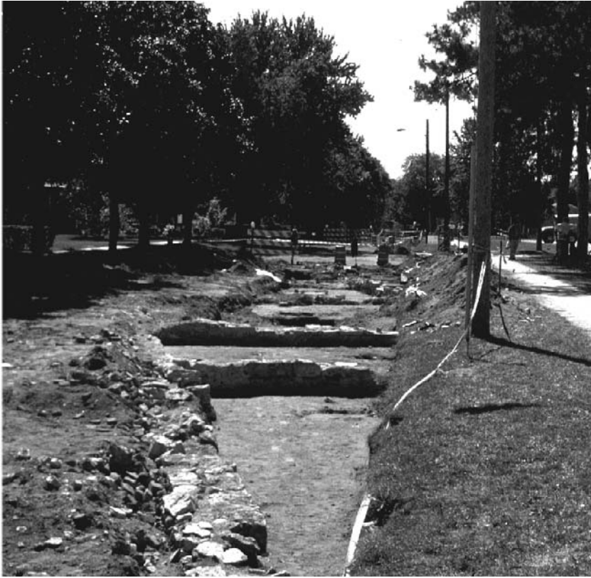
12.3. Stone foundation walls of Second Fort Crawford (1829–1864) being exposed after 140 years beneath Beaumont Road in Prairie du Chien.
