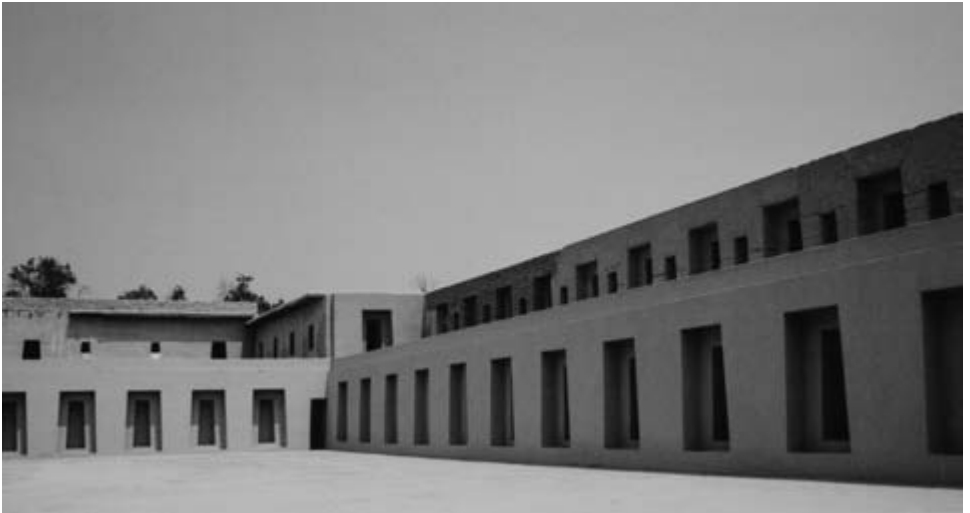
3.8. The Mamacona complex at Pachacamac, Lurin Valley, excavated and restored by Tello. Photo: Richard Burger.
