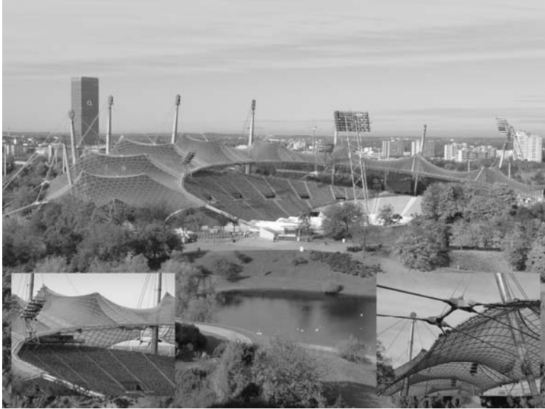
Figure 10-2: The Munich Olympic Stadium of 1972. The roof resembles the Bavarian Alps and is supported by just a few pillars. The two smaller inserts cover details of the construction of the glass-covered cable-net structures (photography taken by the author in November 2012).
