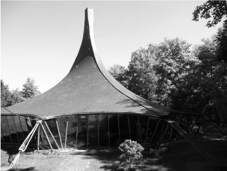
Figure 10-1: Building of Frei Otto's institute at the University of Stuttgart in Stuttgart-Vaihingen. This construction served as a test case for the German pavilion for the Expo 67 in Montral (photography taken by the author in August 2012).
