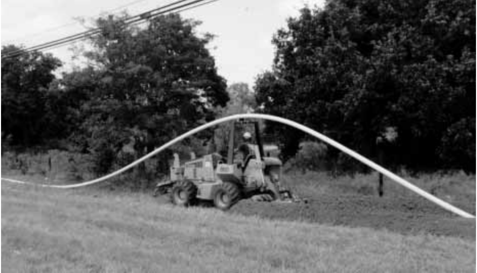
Figure 15-1 Fiber optic cable is often installed in conduit for outside plant applications.
