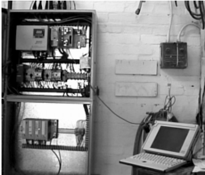
Figure 1.4 A PLC system is housed in a cabinet, shown here with the door open. It controls the resin production plant illustrated in Fig. 1.2. The PLC controller is the small box mounted at the top left of the cabinet, with its control keys situated below its LED display. The low-voltage power supply is mounted to the right of the PLC. The input and output interface units are mounted on the rack below the PLC. Each may be connected to up to eight sensor or actuator devices. On the right is a laptop PC being used for writing programs and downloading them into the PLC. (By courtesy of Kronospan Ltd., Chirk)
