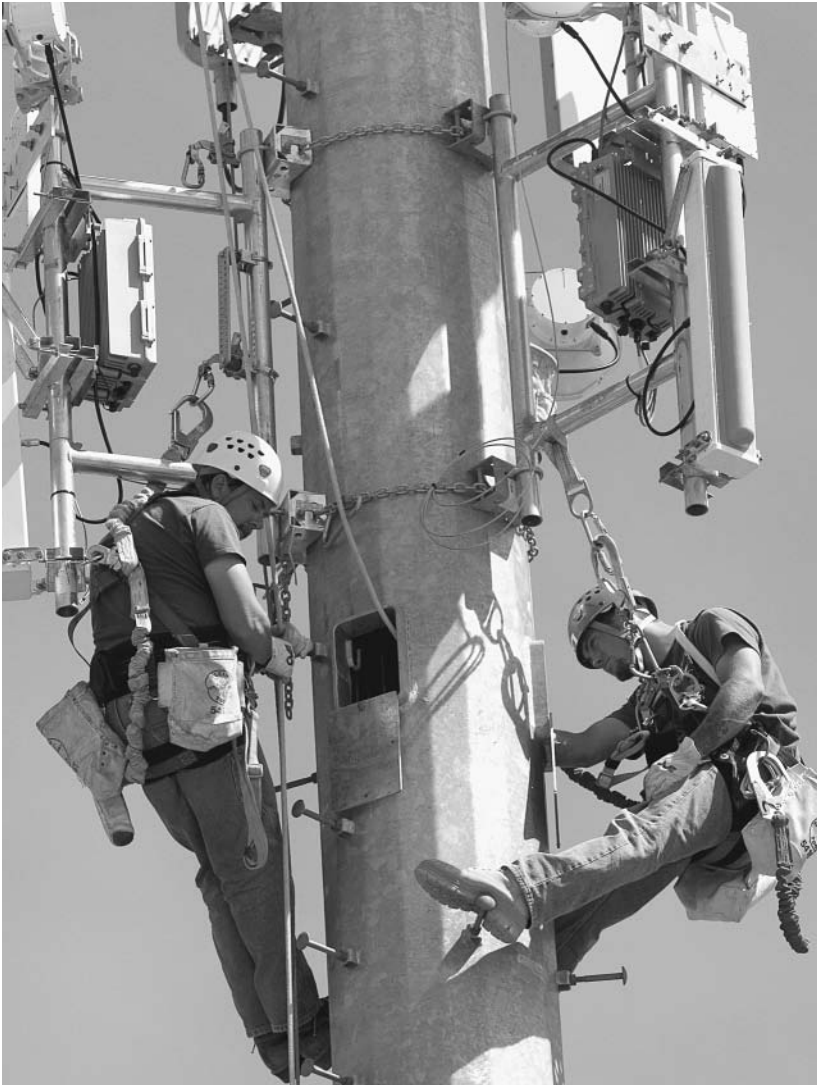
Wireless service technicians repair a cell phone tower. (David R. Frazier, The Image Works )
