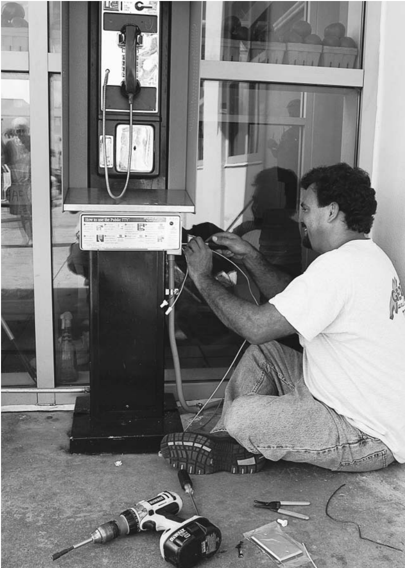
A technician installs a telecommunication device for the deaf on a pay phone. (Jeff Greenberg, The Image Works )
