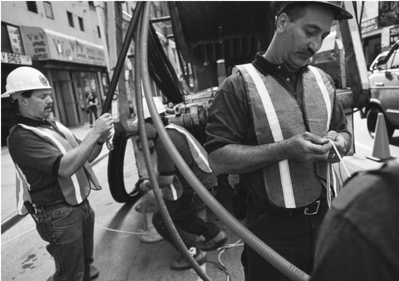
Technicians lay fiber optic cable. (James Leynse, Corbis)
