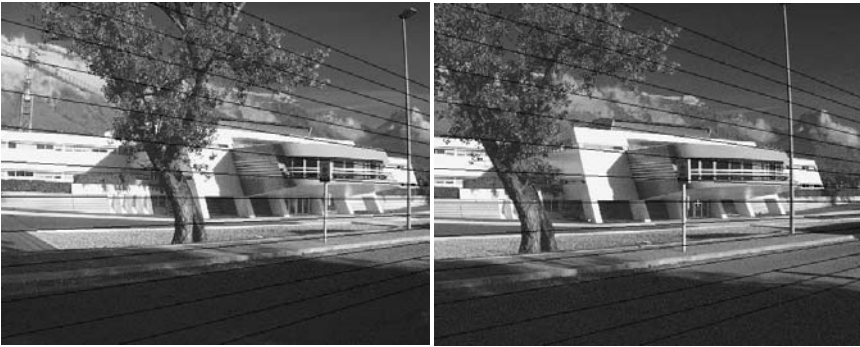
Figure 5.2. Estimation of the epipolar geometry of two images of the INRIA building in Grenoble
