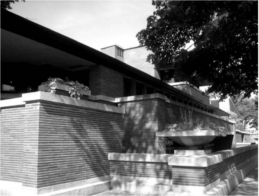
Figure 11.4 Frank Lloyd Wright, Robie House (1908–10). Photograph by the author
