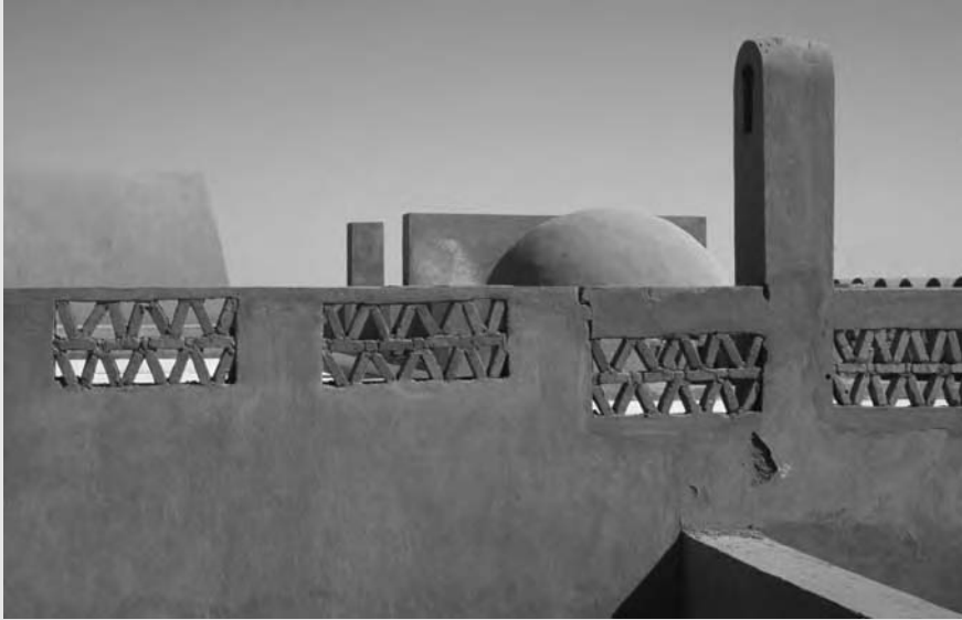
Figure 1.1 New Bariz, Egypt, planned and designed by Hassan Fathy (1965–67), market and agricultural co-operative building (photo M. Miles)
