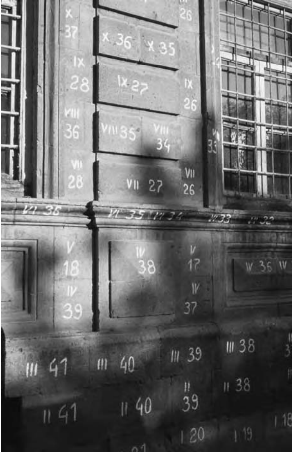
Figure 7.1 Yerevan, building on Republic Street prepared for removal (photo M. Miles)
