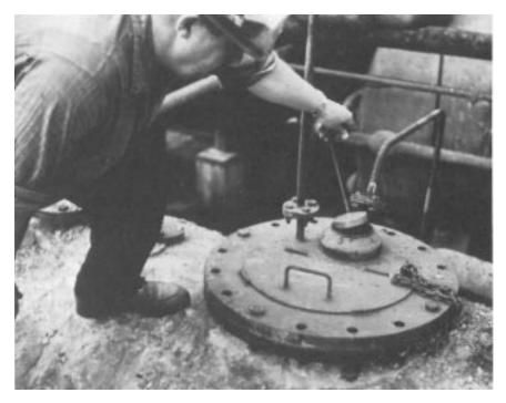
Figure 7.3 The flame trap assembly, showing how the flame trap can be removed for inspection
