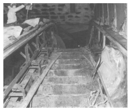
Figure 18.1 The top of the escalator at King's Cross after the fire. (Reproduced by permission of the Health and Safety Executive.)
