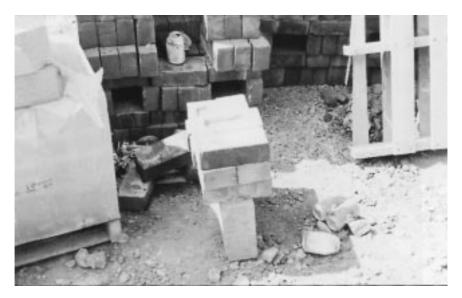
**Figure 22.1** Reconstruction showing how the brick columns were supported on lightweight blocks (Reproduced with the permission of The Controller of Her Majesty's Stationery Office)
