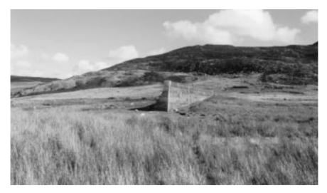
Figure 22.2 Part of the Llyn Eigiau concrete dam today. The broken end has been straightened
