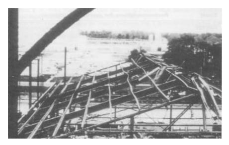
Figure 4.2 The result of an explosion in a hydrogen compressor house
