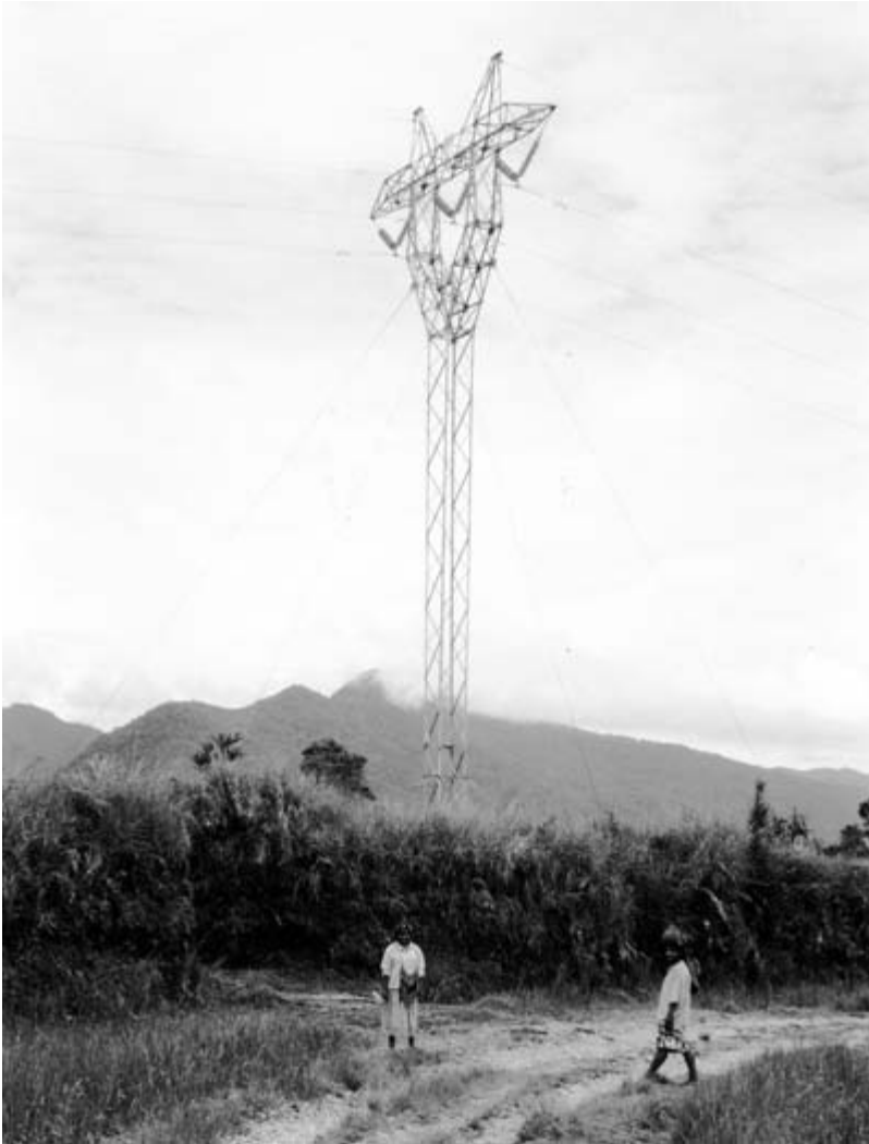
FIGURE 4. One in the chain of pylons that threads up and down mountains and through people's gardens, carrying electricity from the Hides power station south of Tari to the Porgera gold mine in Enga Province. Disgruntled landowners occasionally topple these pylons, shutting down Porgera for days or even weeks at a time.
