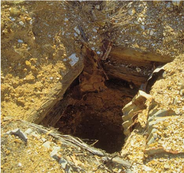
Fig. 35. Unsecured, open shaft in the abandoned Coolgardie/Australia gold mining field.
