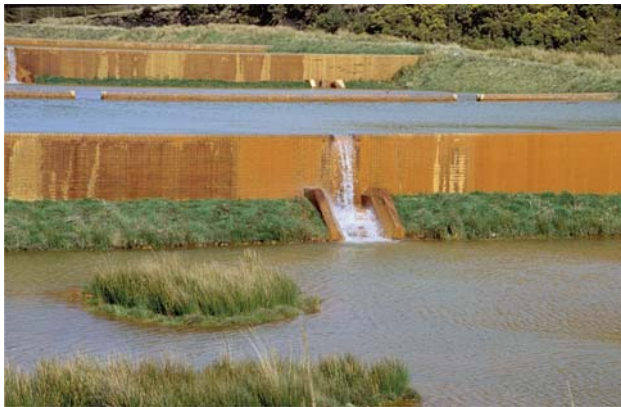
Fig. 91. Mine water overflowing the Pelenna II/Wales system. The hydraulic head is too low to drive the water through the compost (24 March 2000).
