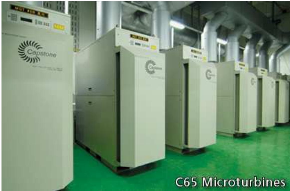
Figure 2. Capstone microturbine, model C65 (Capstone, 2012).
