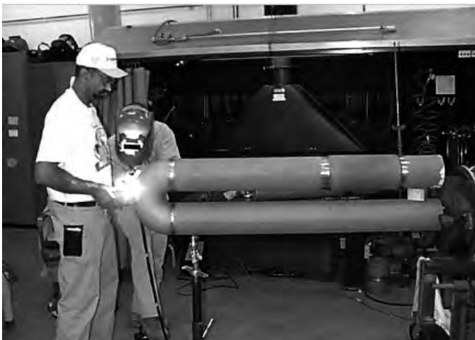
FIGURE 5.9 Radiant burner tube.
