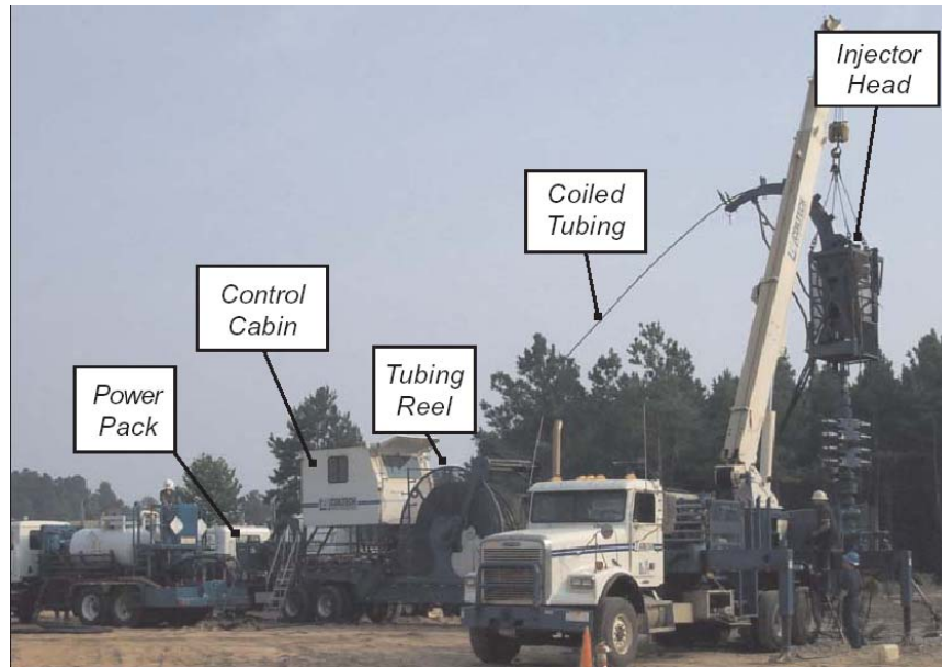
Fig. 2.1—Trailer mounted CT unit and crane. 1
