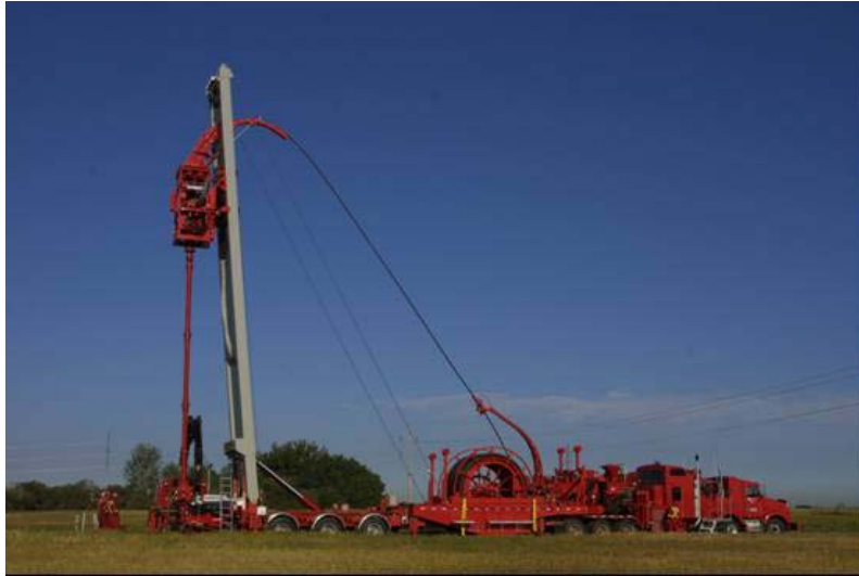
Fig. 2.2—A coiled tubing mast unit is rigged up. †
