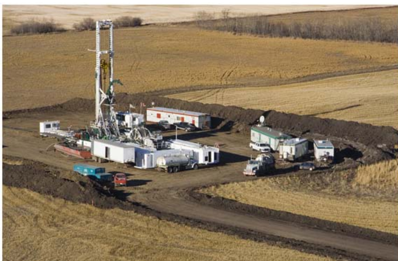
Fig. 2.6—Coiled tubing drilling wellsite. §
