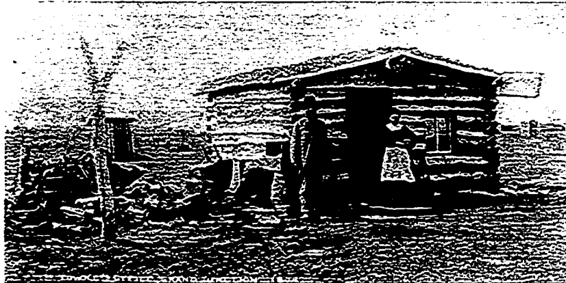
Figure 4 First Town Company Building 59
