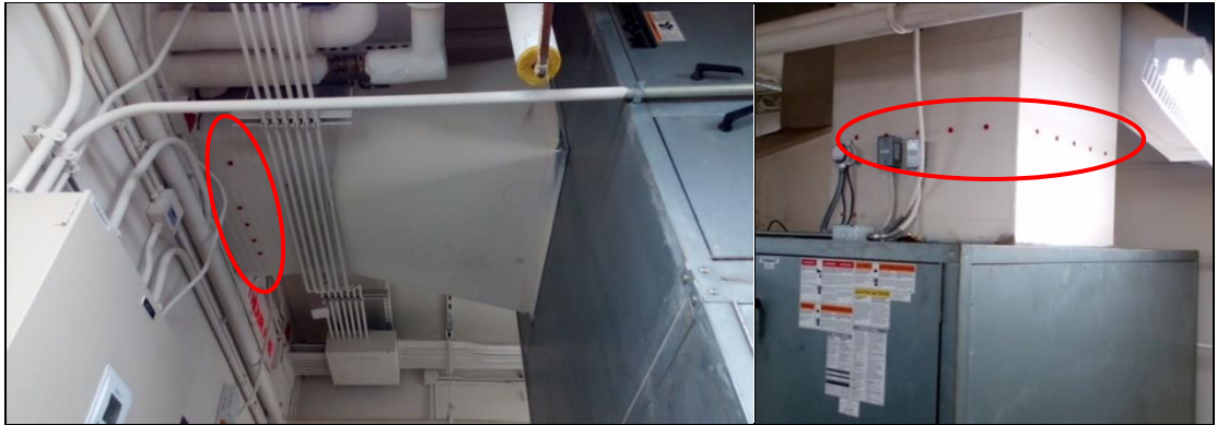
Figure 2-7: Typical placement of holes for TAB procedures.
