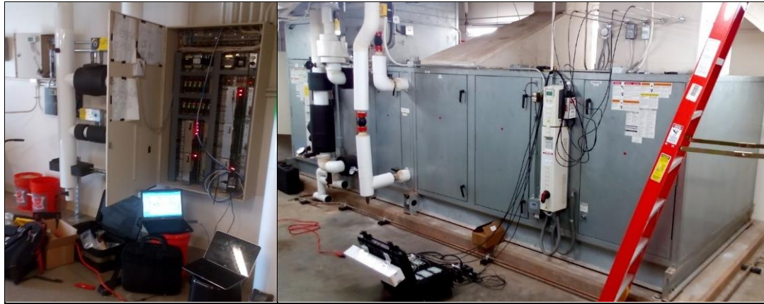
Figure 2-11: Testing set-up for performing in-situ airflow measurements.
