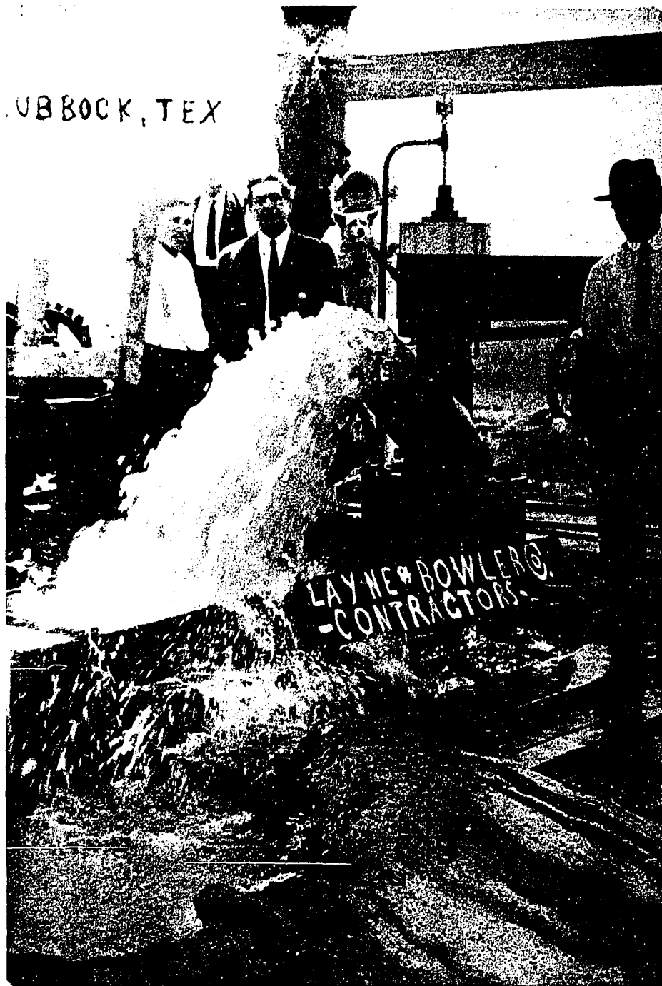
"PIT-LESS" PUMP IN OPERATION. A LUBBOCK IRRIGATION COMPANY WELL NEAR LUBBOCK, TEXAS, IN 1913
