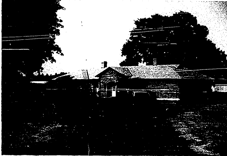
Fig. 29--One of the community buildings at Sabine Farms, note how well the building is maintained.
