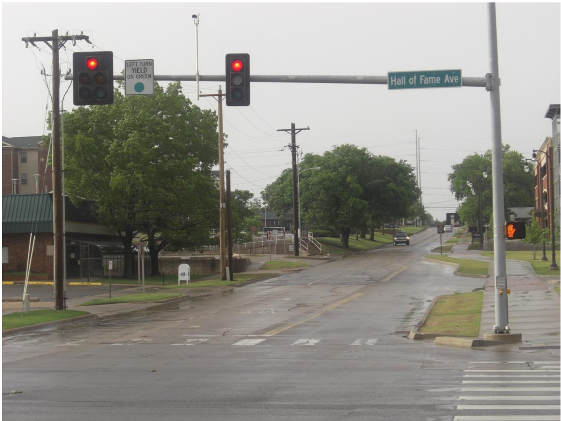
Figure 1-1: Cantilever sign support structure
