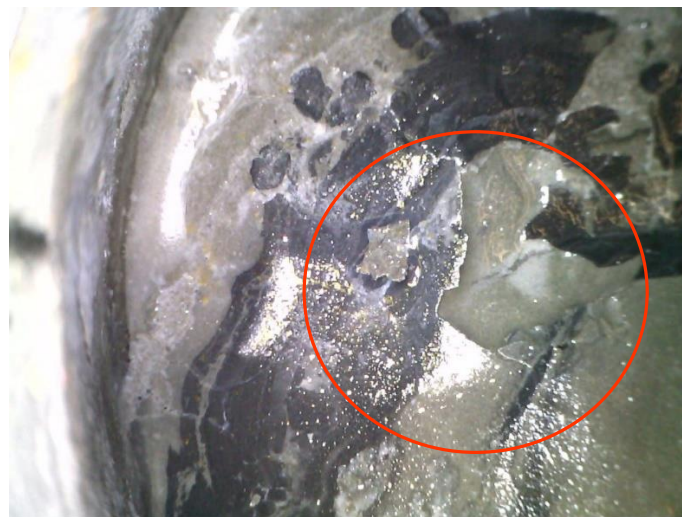
Figure 66: Nanomaterial Cement Sample with leak position highlighted in red.
