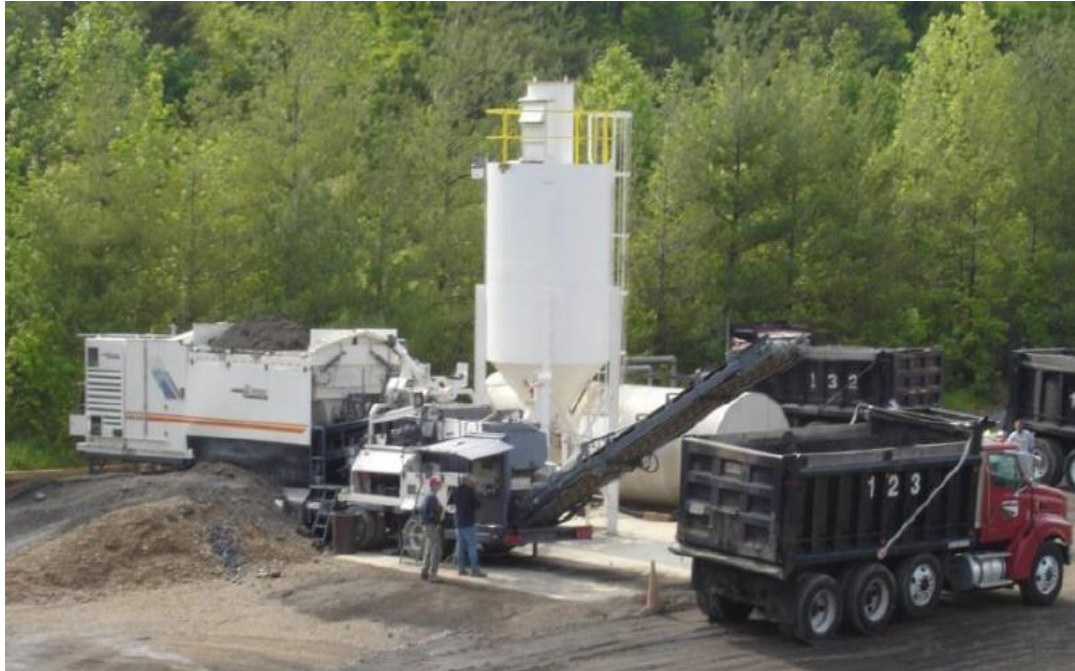
FIGURE 4 Cold Central Plant Recycling (7)
