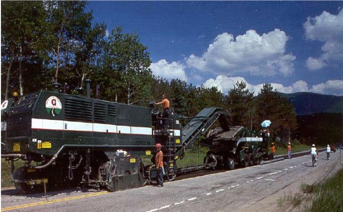
FIGURE 2 Two Unit Recycling Train
