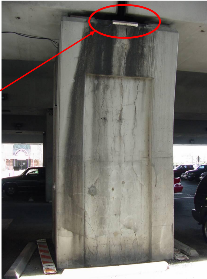
Fig. 4.1 Supporting column of the bridge
